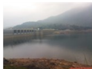
KMTR-Ambasamuthiram Servalar Dam
